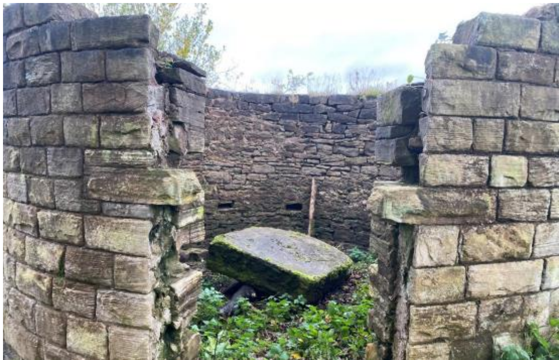
Photo 6: Derelict building to be converted
